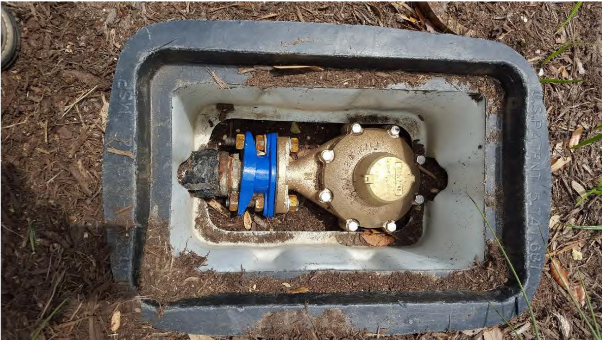
Photo 8 – Cycle 17 Meter at 134 de oro (tight fit for new 1.5-inch meter; meter box would be removed during meter replacement and should have been upsized):
