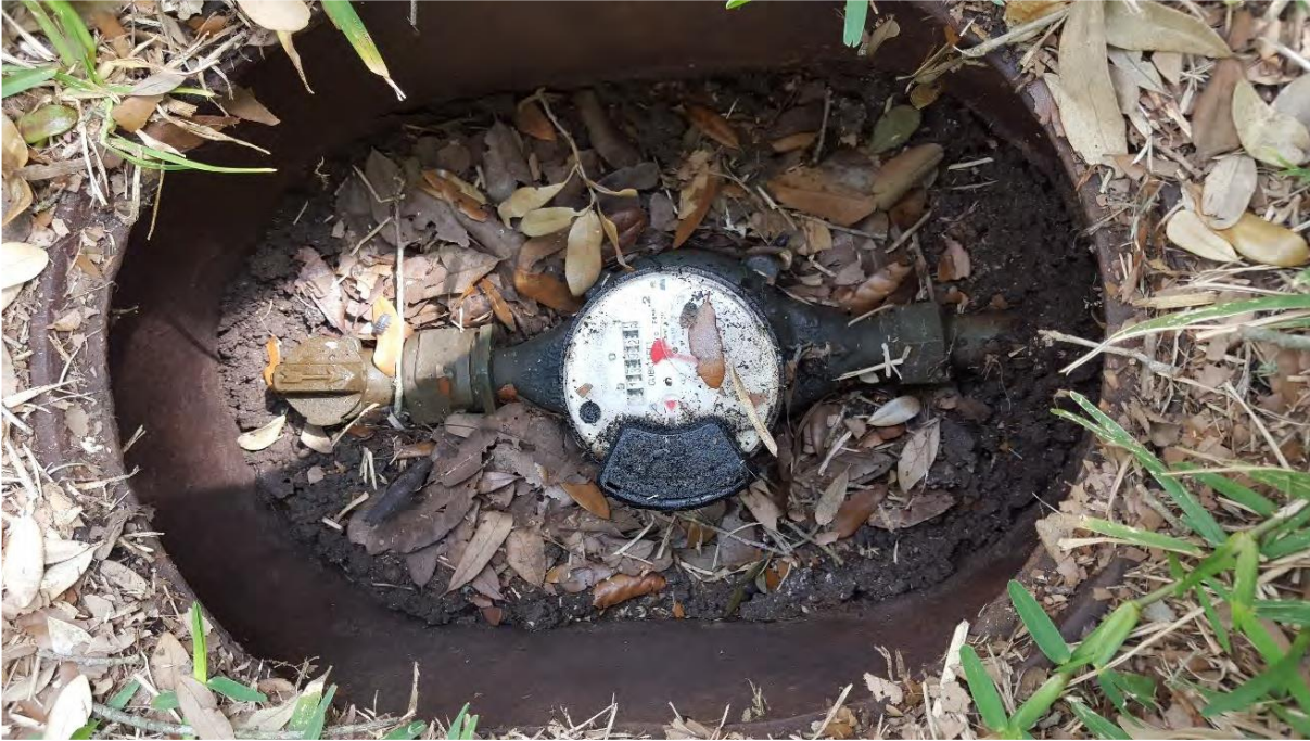
Photo 1 – Cycle 6 Meter at 106 Castle Oaks (requires meter box clean-out):
