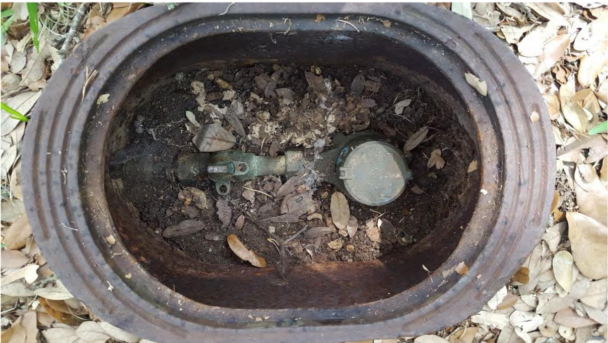
Photo 2 – Cycle 6 Meter at 106 Wisteria (may require meter box removal for new meter installation due to meter being offset in box):
