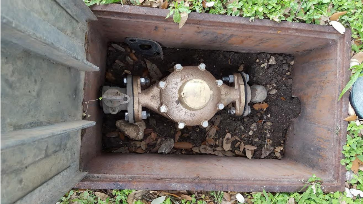
Photo 4 – Cycle 6 Meter at 4331 Vance Jackson (tight fit in existing meter vault for new 1.5-inch meter):
