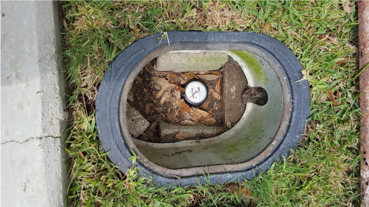
Photo 14 – Cycle 17 Meter at 1525 Keats St (clean out excessive dirt/debris in meter box; add meter yoke to raise meter closer to grade):
